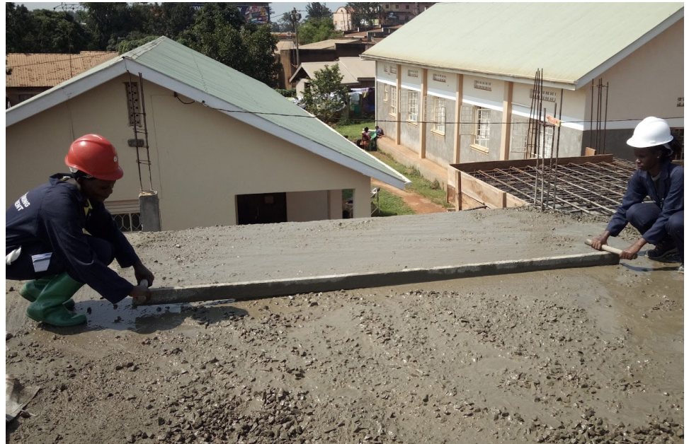
Figure 1: Graduate interns on site levelling concrete
